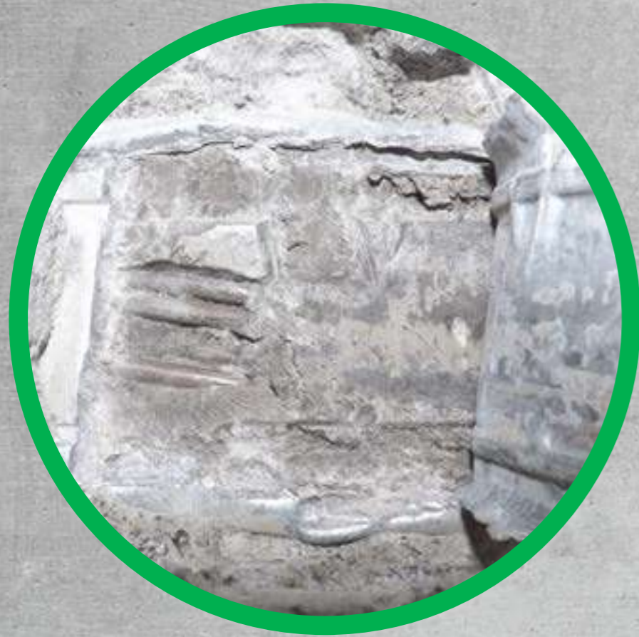
Properly Grouted No Corrosion
