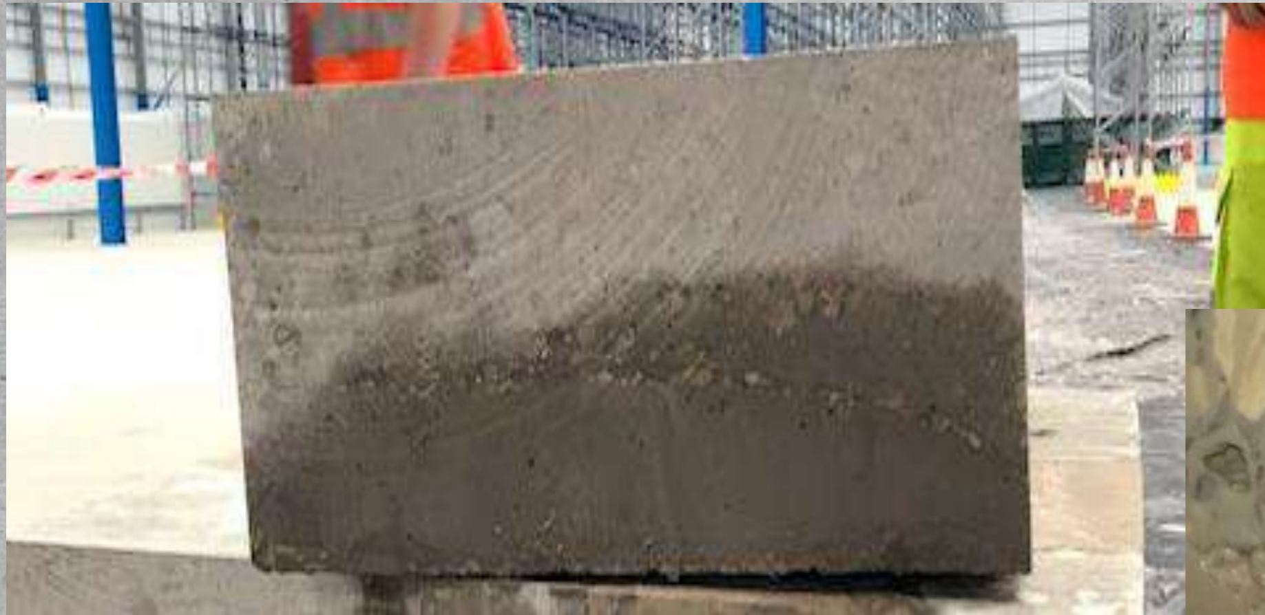
Formed SWF Concrete
