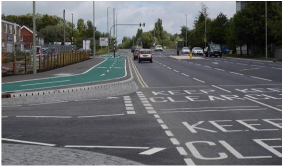
Completed Gloucester South-West Bypass Scheme
