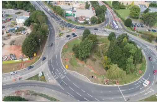
Completed Arle Court Roundabout
