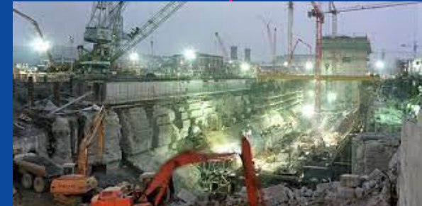
9 Dock Upgrade – the last major construction in Devonport
