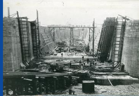
Dock construction 1900's
