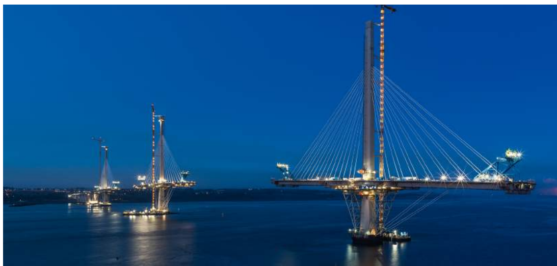
Figure 20 (c): The Queensferry Crossing under construction
