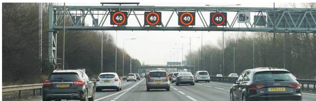
Figure 22: A smart motorway section of the M60 with all lanes running
